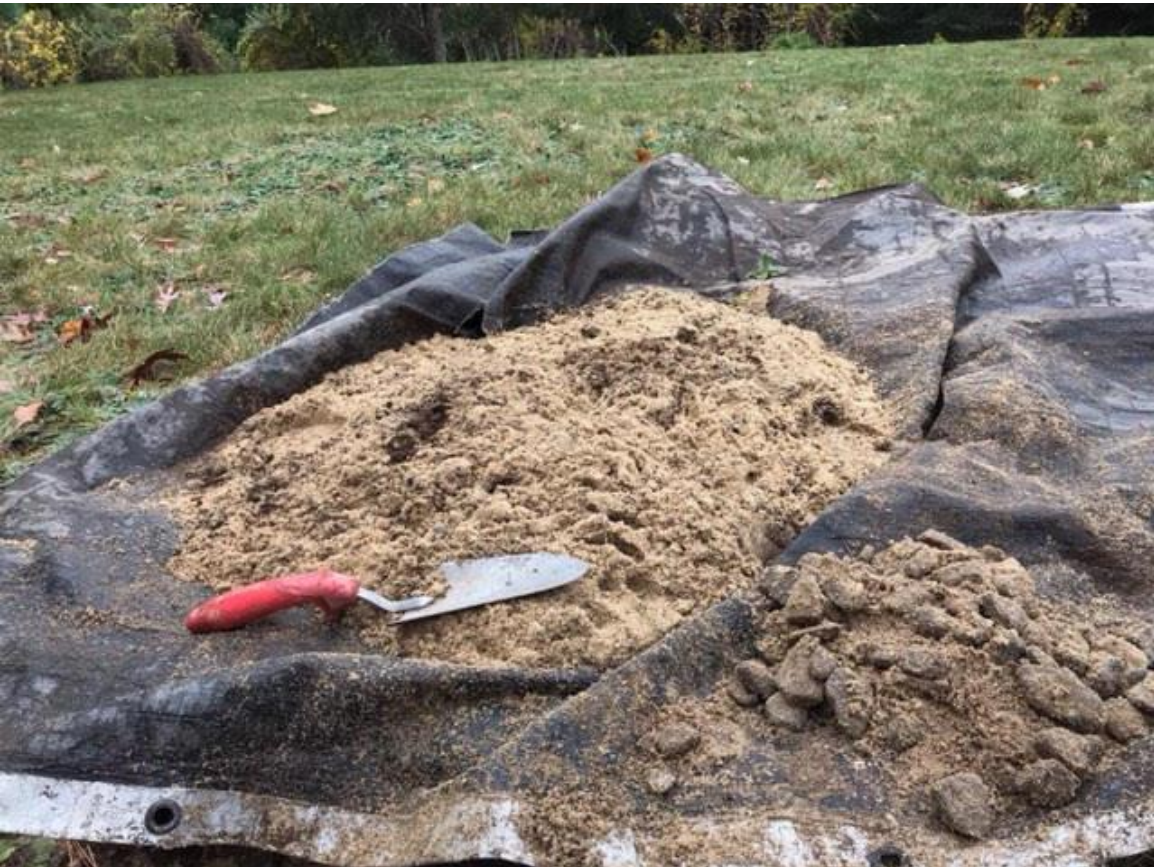
FIELD C – Observation hole #2 sand and stone
